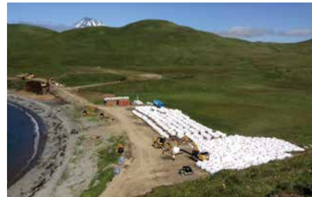
Nikolski cleanup of contaminated soil from WWII by crew from Cape Environmental. Each container can weigh up to 2,200 lbs. and must be lifted by crane and loaded onto a barge for removal. —Photos by Vincent Lestenkof.
